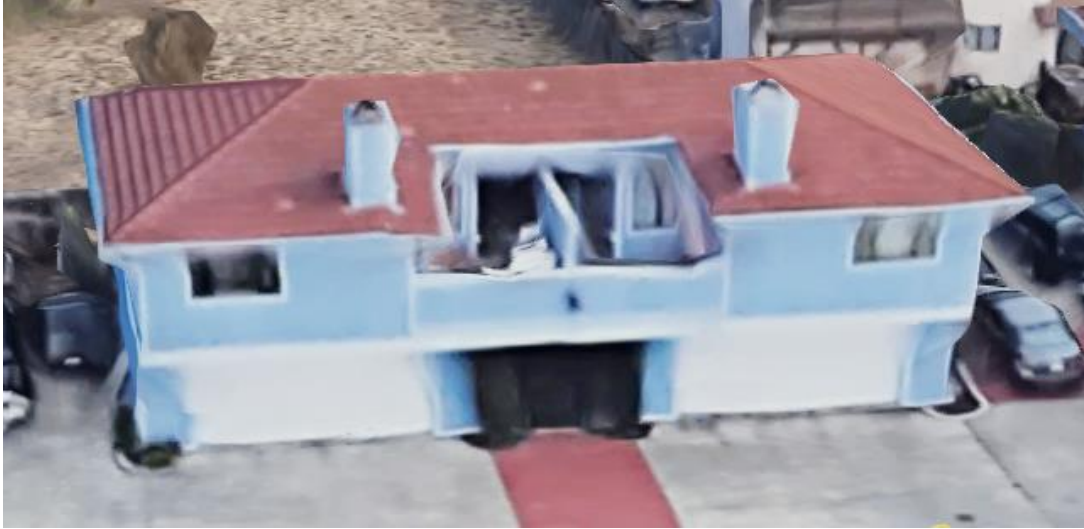
Figure 7: Hayward Apartments 3 and 4
