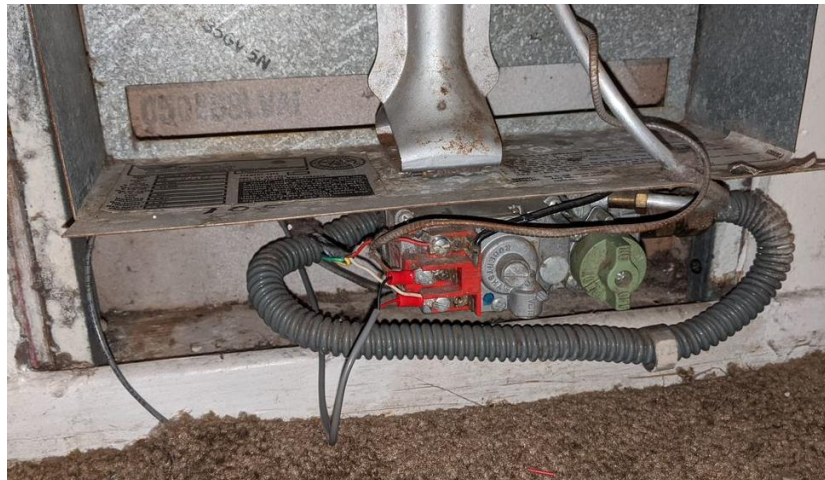
Figure 2: Sample Wall Furnace Voltage Bridge Wiring
