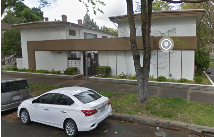
Figure 10: Sacramento Multifamily Apartment Building
