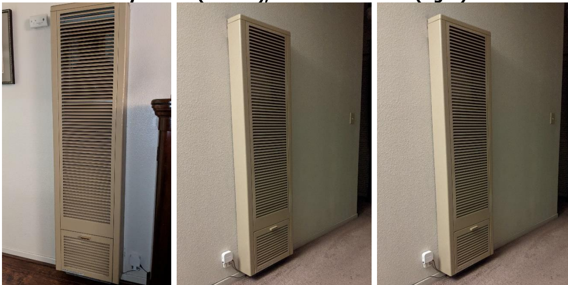
Figure 4: Existing Baseline Wall Furnaces in Hayward 3 (left), Hayward 4 (middle), and Oakland SFH (right)
