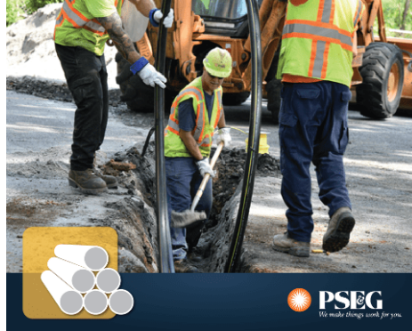
Gas System Modernization Program WORK PHASE 2 – Install New Pipes
