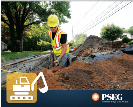
Gas System Modernization Program WORK PHASE 1 – Dig Trench
