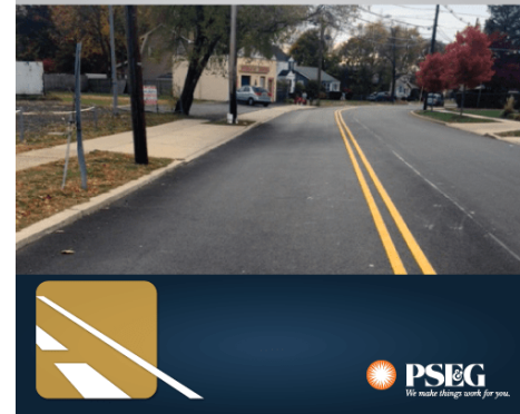
Gas System Modernization Program PHASE 4 – Final Road Restoration
