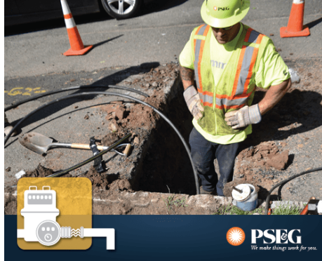
Gas System Modernization Program WORK PHASE 3 – Connect Service Lines
