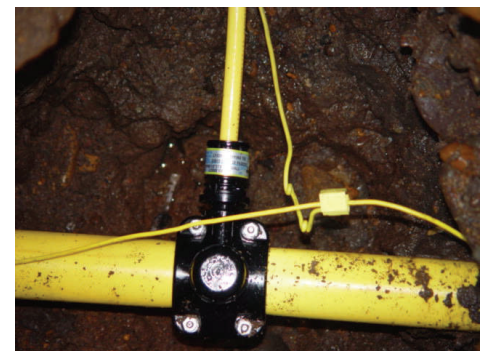
Tracer wire connection
