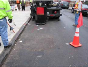
1. Coring unit with conventional repair in foreground.
