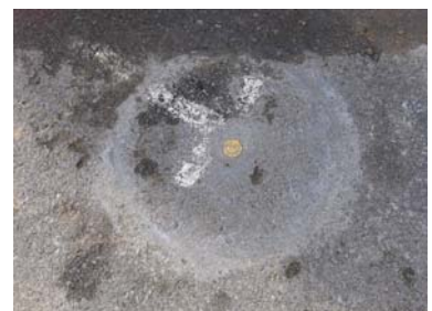
10. Reinstated core—almost invisible
