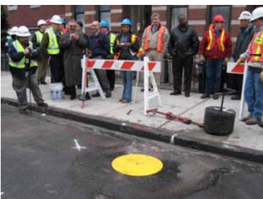
4. Temporary road plate
