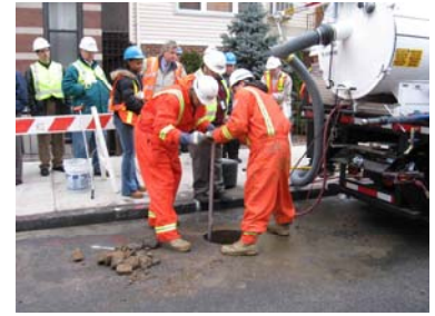
6. Turning off the gas
