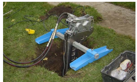
Below: Small footprint excavation
