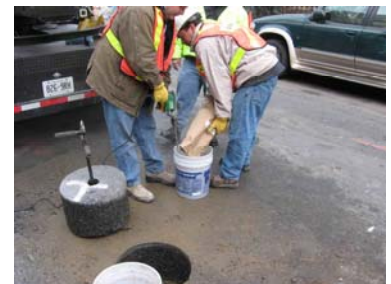
8. Mixing the Utilibond
