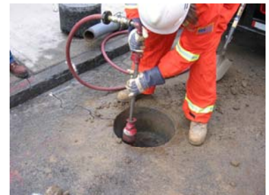
7. Compaction (note wire from Soil Compaction Supervisor)
