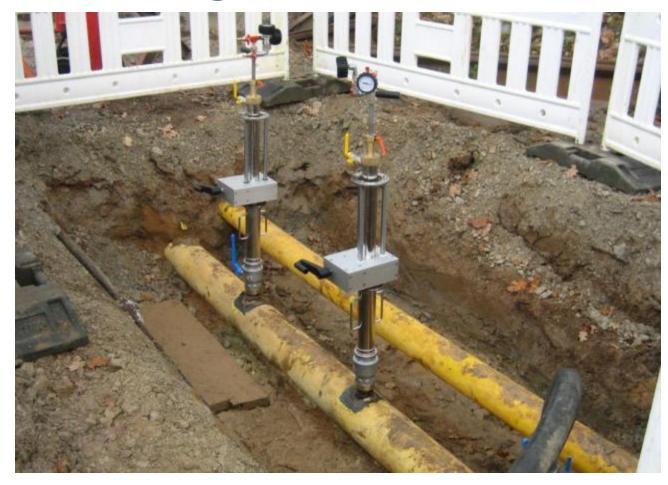
> Flow stopping 2"- 8" operating at pressure up to 60 psig
