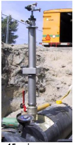
> Flow stopping 3"- 16" operating at pressure up to 15 psig
