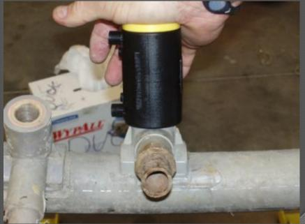
THE INSERT HOLDING TOOL SHALL BE USED AT THIS TIME PRIOR TO FUSION OF COUPLING AND INSERT TO THE ALDYL-A TAPPING TEE.
