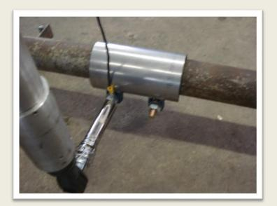
Some procedures demand that an anode be attached to hardware that has been added to the main.
