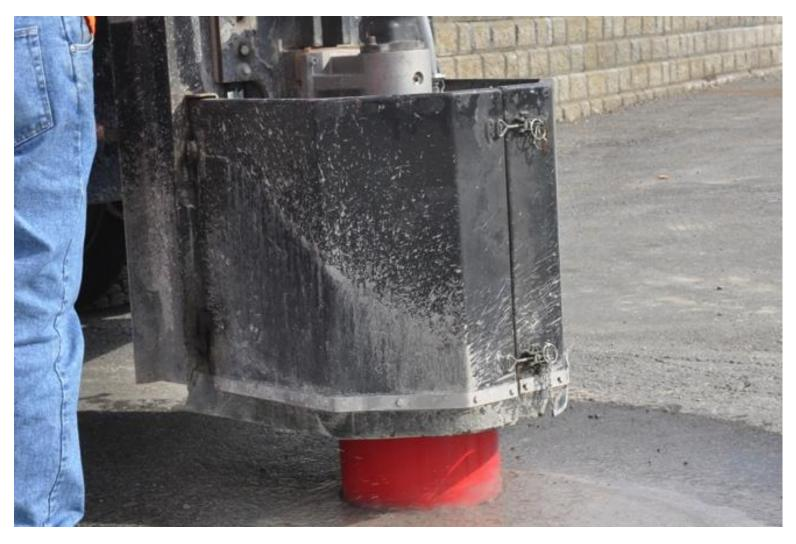
Core 12" hole through pavement around existing valve box (remove pilot pit) or location of test station.
