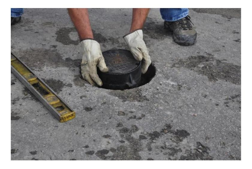
Add 1-2 inches of pea stone and install test box or new valve box.
