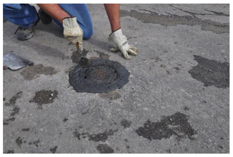
Consolidate the mixture into the hole to make sure there are no voids. If the Utilibond mixture is slightly below the surface add pea stone to mix and consolidate again.
