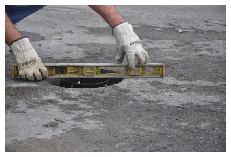
Using a straight edge make sure the top of the box is flush with the surrounding pavement.
