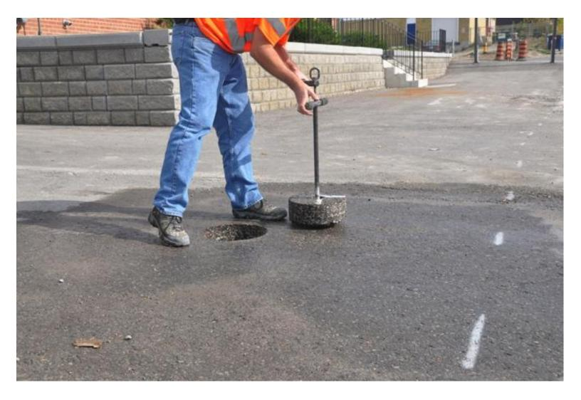
Remove core with core puller and or sunken valve box by hand. Clean up area.
