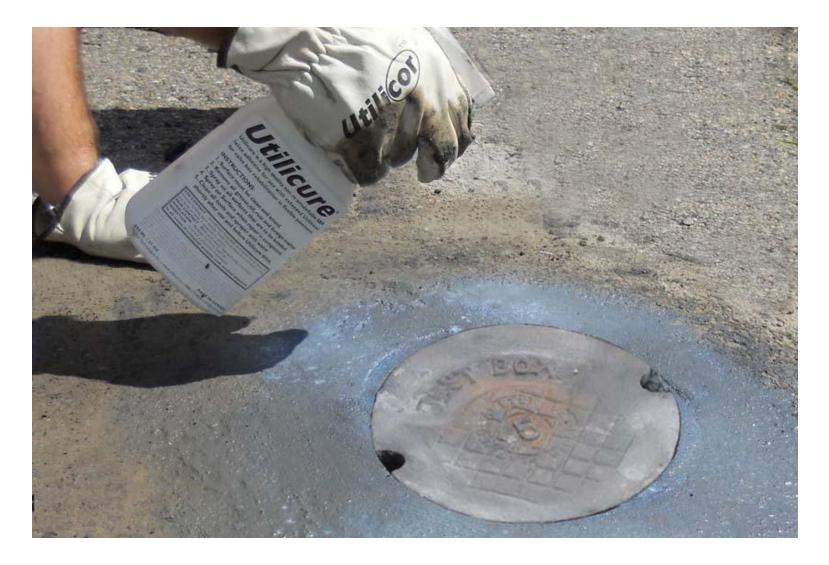
Spray surface with Utilicure to ensure proper hydration and Prevent surface cracks.
