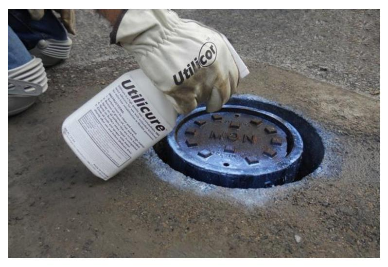
Generously spray all areas to be bonded, on valve box and pavement with Utilicure. Do not allow Utilicure to dry, if it does reapply.
