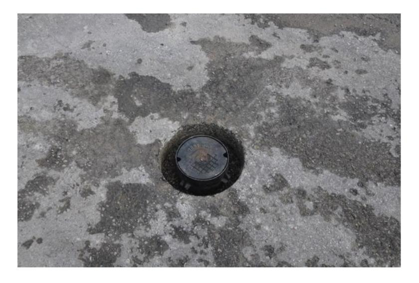
Test box or valve box is flush and ready.
