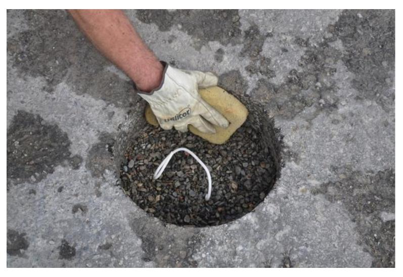
After test wire is installed and hole is back filled and compacted to about 2 inches below base of pavement or 6 to 8 inches below the surface clean the sides of the pavement.
