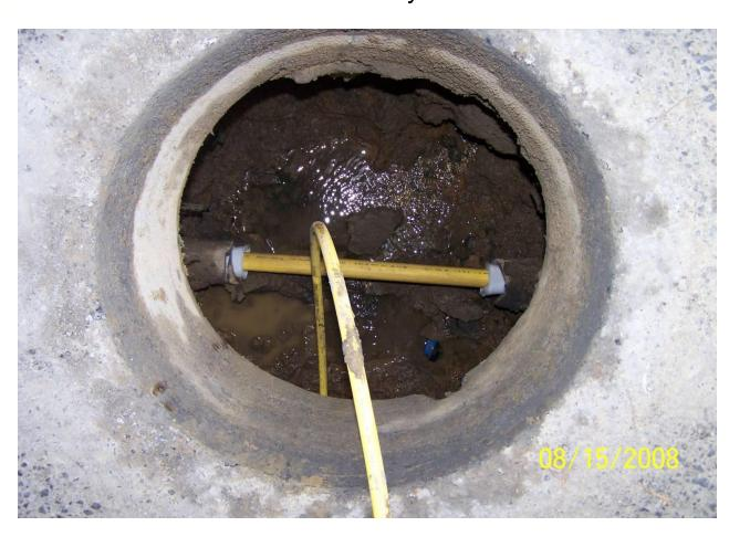
Preparing to Install Electrofusion Tee with Extension Tool
