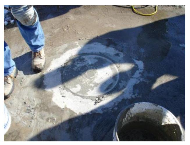
Because temperature of core and hole approx: 60°F at end, Utilibond strength gain time approx: 40 minutes.
