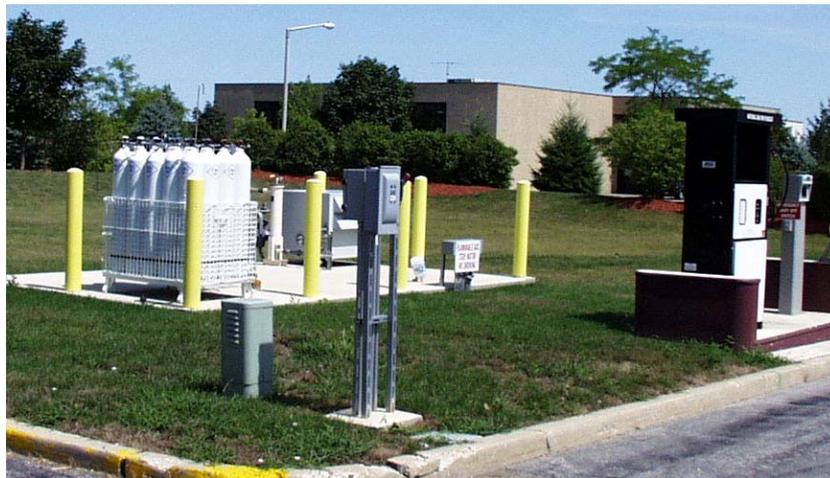
**Figure 3: Three Bank Cascade With Multiple DOT Vessels**
