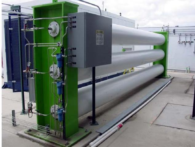
**Figure 2: Three Bank Cascade With ASME Vessels**
