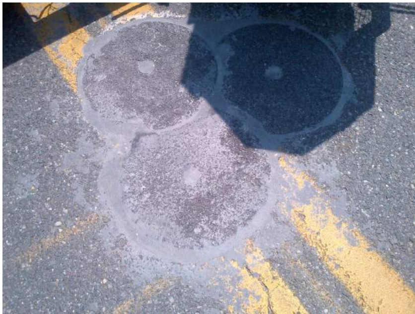
A triple core cut, extracted, and reinstated as one repair
