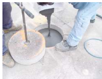
Utilibond™ poured into hole
