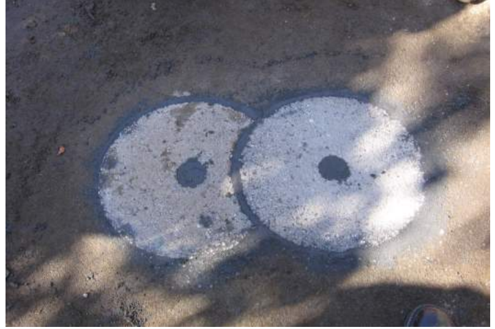
Two cores that have been simultaneously reinstated
